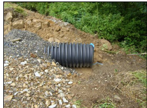
Newly installed culvert pipe under Mottarn road
