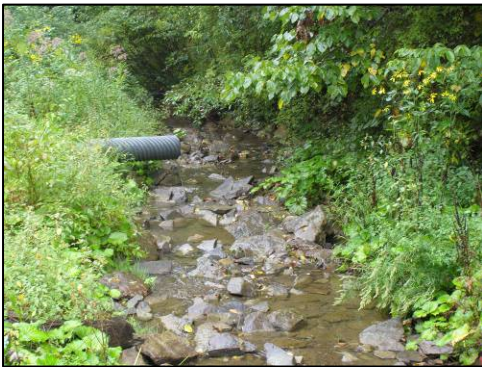
Stormwater pipe that enters into Hays Run
