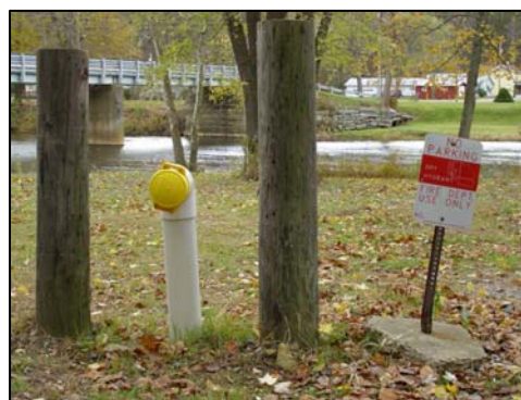
Dry hydrant located at Putneyville Park is used by firemen needing access to water in emergency situations where there is no public water system and a lack of fire hydrants
