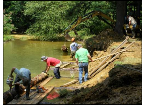
WPC and volunteers installing streambank stabilization and habitat structures on a tributary to Little Mahoning Creek
