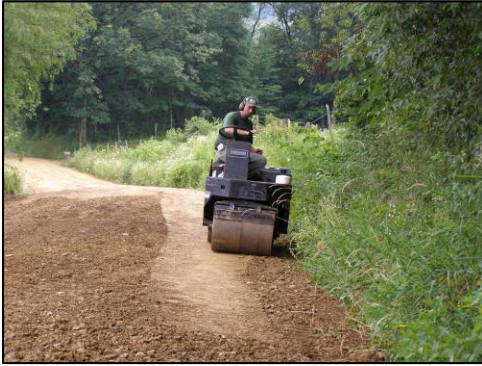
Mottarn road dirt and gravel road project during construction phase in July 2008, where 11 culverts were installed and the roadway was re-graded
