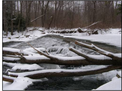
Savan Dam located on Little Mahoning Creek in Grant Township, Indiana County
