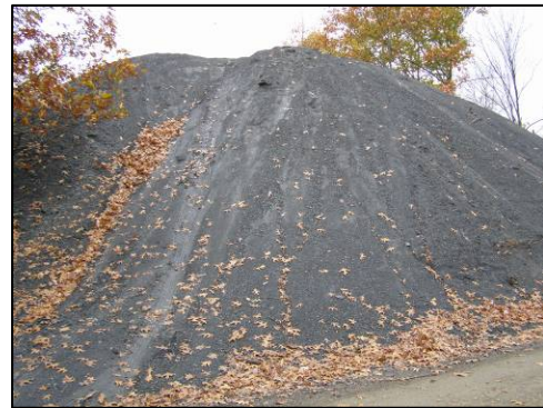
Refuse pile located in the Pine Run watershed where coal formed in the Conemaugh and Allegheny formations was mined
